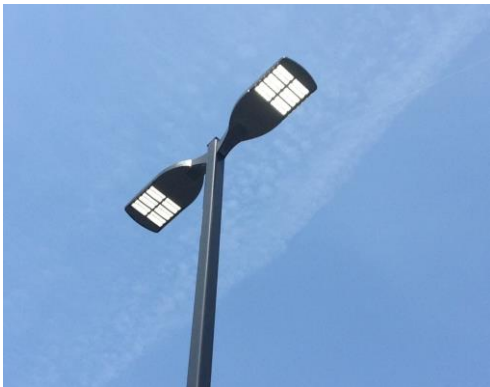
Downcast area lighting (parking lot or roadway)
